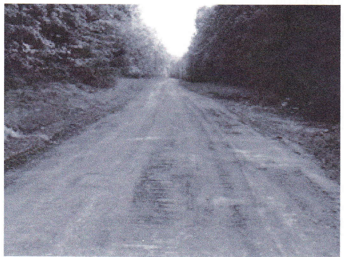
This is a view of the widened road bed.
